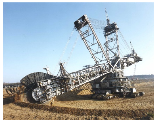
Fig. 5: "Drive system" bucket wheel excavator
